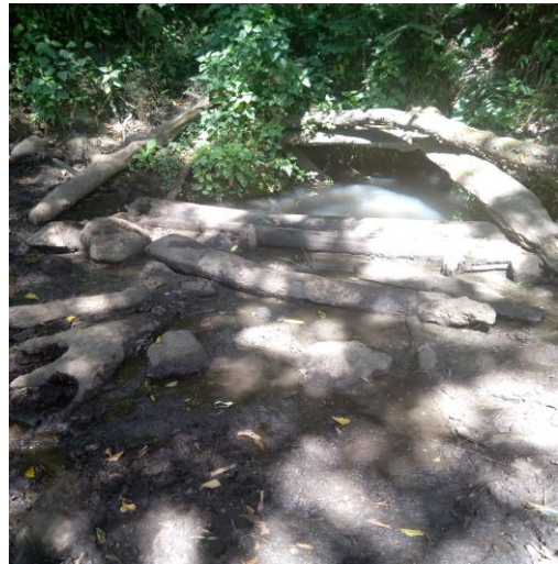
Plates 4.2: Photographs of the two semi-protected springs are fenced off with either a stone wall or wood plugs to keep away large animals (Source: field data)
