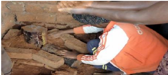
Figure 3: Building edges and combustion chambers
