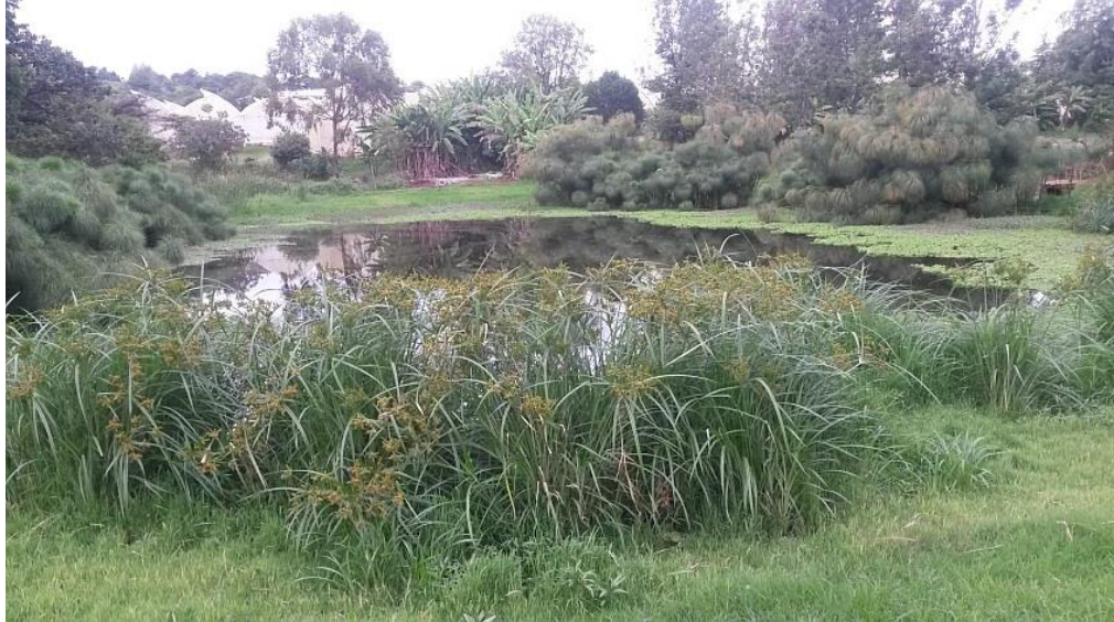
Plate 4.4 Horizontal sewage treatment wetland in Karen Golf and Country Club
