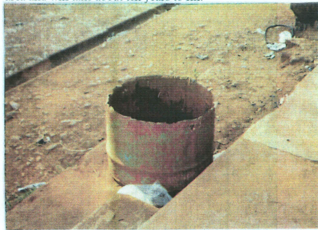
Plate V: A waste storage facility at a commercial premise in town. Notice the rust, and the sharp rough edges that could pose danger to waste handlers.
