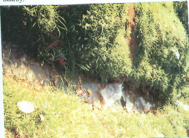
Plate IX: A drain clogged with wastes such that water remain stagnant thus creating conducive conditions for breeding of disease vectors such as mosquitoes and flies.
