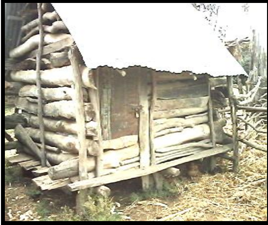
Plate 4.1e: Wooden iron roofed granary the for maize sotrage
