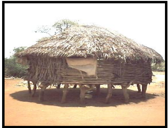
Plate 4.1b: Wooden grass roofed granary for maize storage
