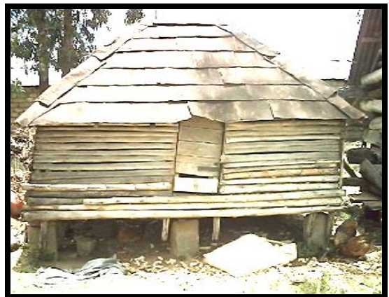
Plate 4.1d: Sisal stalk iron roofed granary for maize storage
