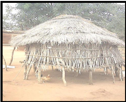
Plate 4.1c: Wooden grass roofed granary for maize storage
