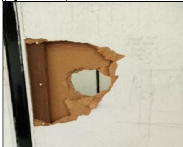
Figure 8: Illustration of a hole through and, scuff marks on a pin-up board at the UON. Source: Kebenei, 2025.
