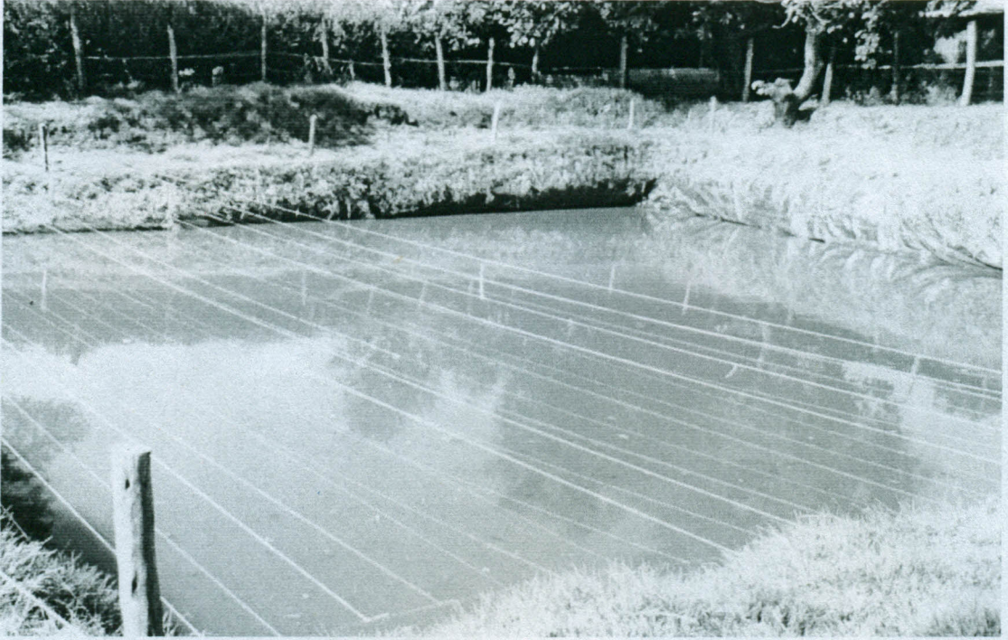
Lined Pond with partial Overhead security and Perimeter Fencing
