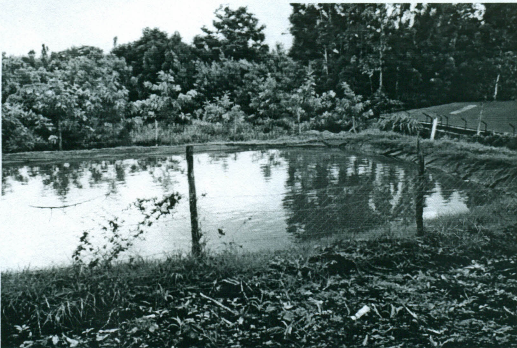
Lined Pond with Perimeter Fencing
