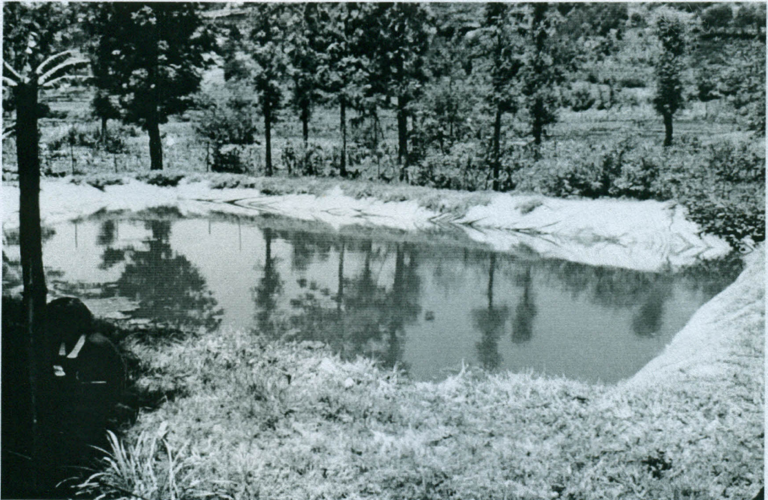
Unsecured Lined Pond
