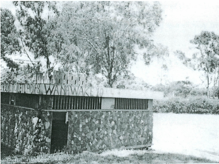
Plate 1: An abandoned toilet under the management of NCC at Uhuru Park
