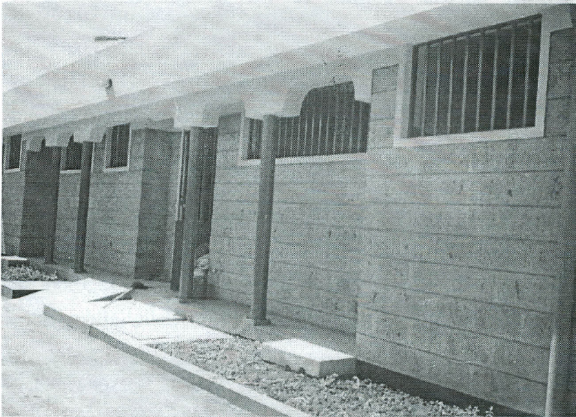
Plate 3: Modified toilet at Railway Station
