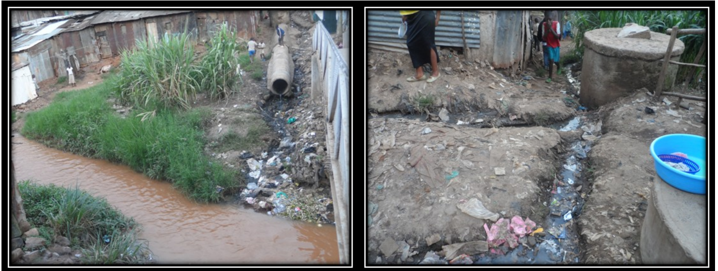
Plate 4: Photographs showing lack of infrastructure within the Mathare settlement
