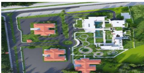
Figure 3: Aerial view of the site. Source: Author, 2024.
