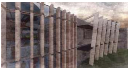
Figure 6: Use of sun shading fins for solar protection. Source: Author generated; 2024
