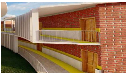
Figure 18: Use of balusters as a safety feature. Source: Author, 2024.
