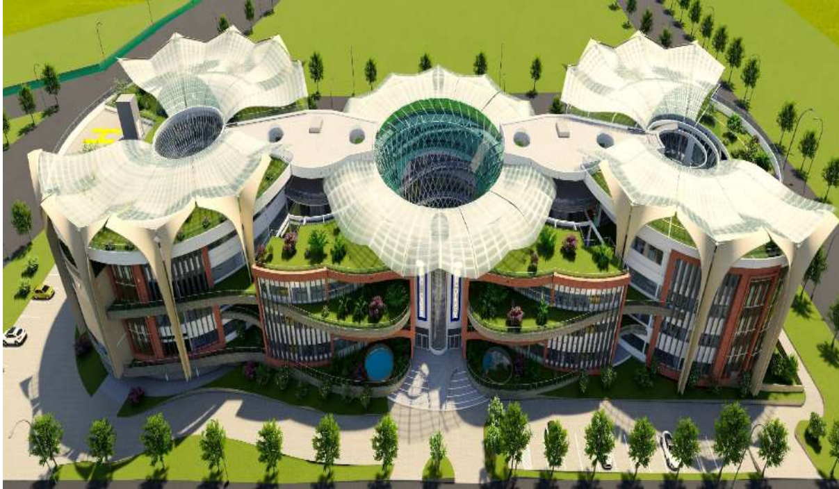
Figure 1: Exterior perspective of the Oncology facility showcasing daylighting atriums, solar tubes, solar harvesting roofing, wind interactive facade louvers and green terraces incorporated as passive design approaches. Source: Author, 2024.
