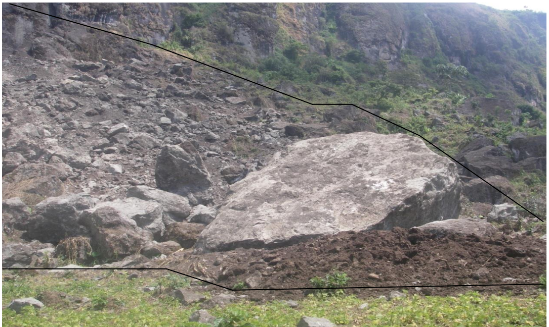
Plate 4.1: Rocks from a collapsed rock face on Wanale scarp (Mbale 2009)
