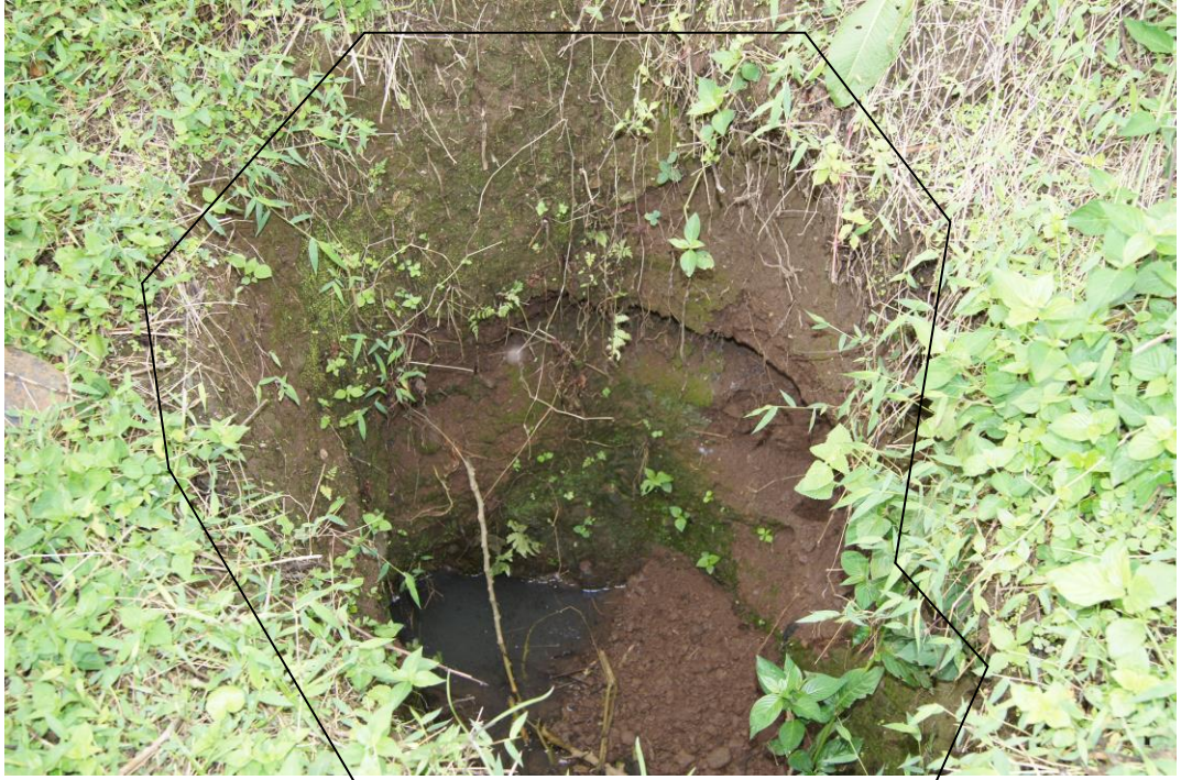
Plate 6.3b: A hole through which groundwater oozed out to the surface (Bukhalasi 2010)
