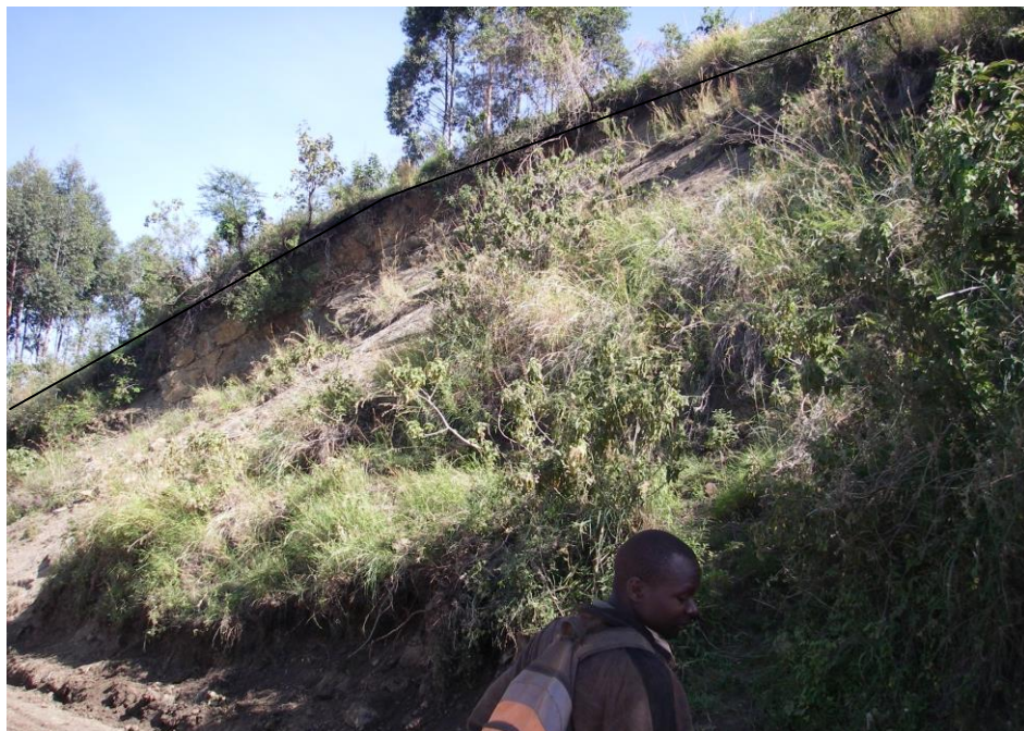
Plate 5.4b: A land slide scar initiated by the road side on the upper convexity of a slope (Bufupa - November 2009)
