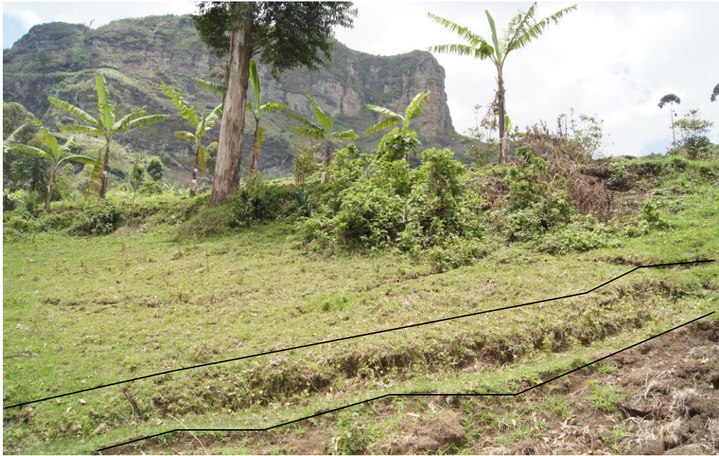
Plate 4.5a: A tension crack cutting across the top of Namisindwa ridge (Buwere 28 th May 2010)
