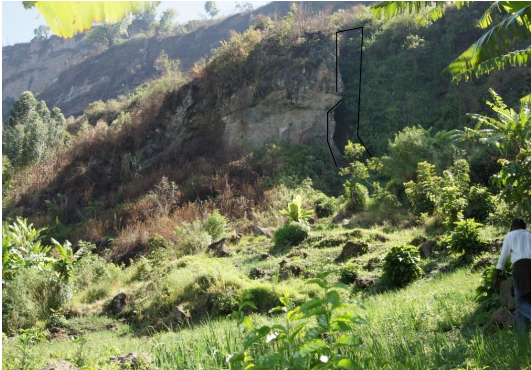
Plate 4.5b: A tension crack cutting through Namisindwa ridge Scarp (Bukwapa 30th May 2010)
