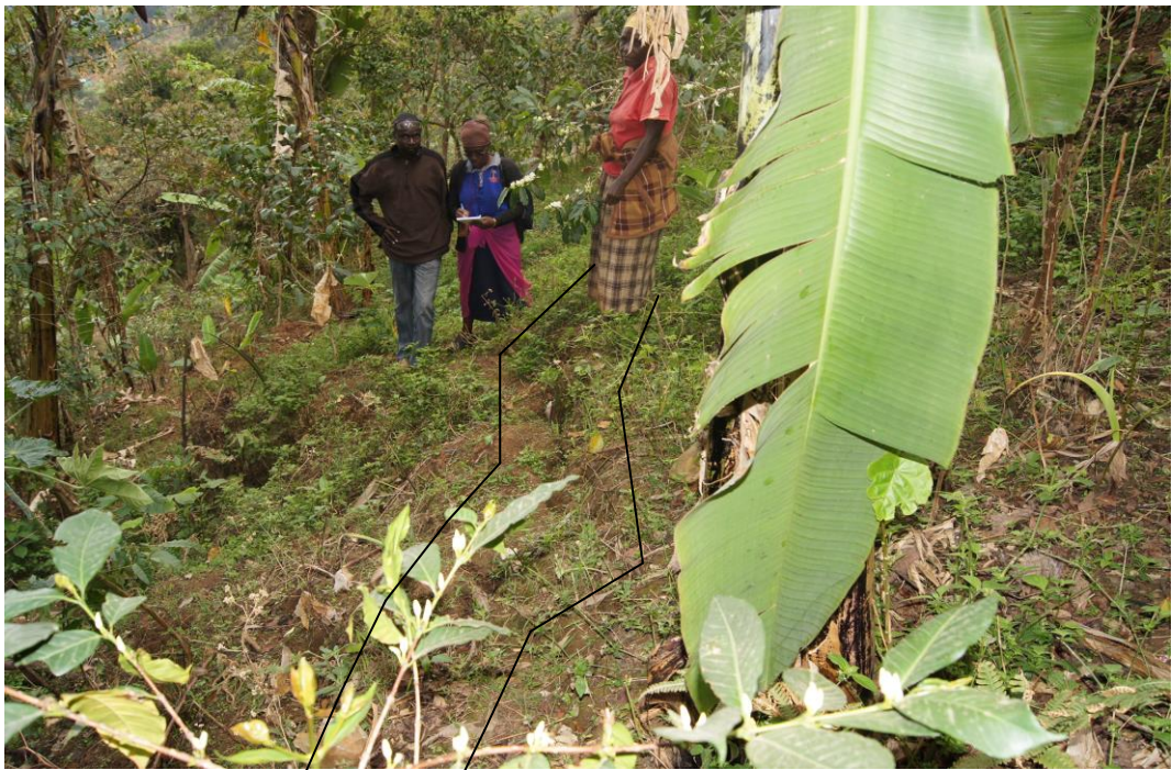
Plate 4.5c: A tension crack cutting across Tsekululu hill (Bunambale May 2010)
