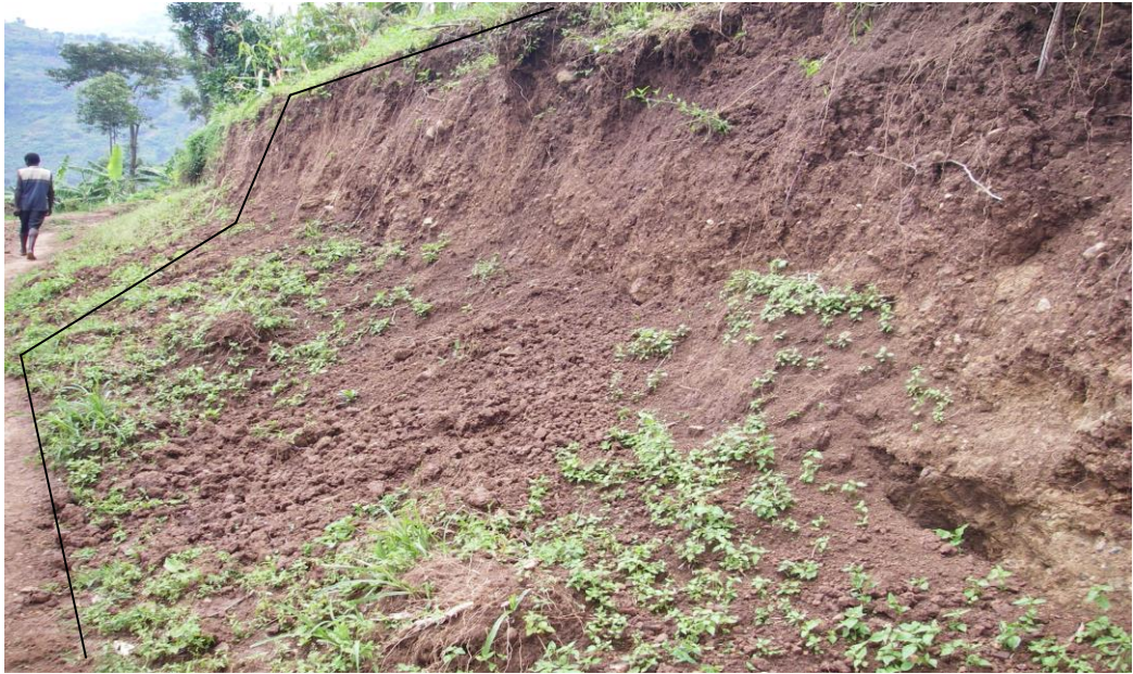
Plate 4.2: An earth fall experienced on a road side cutting in August 2009 (Bufupa 24 th November 2009)
