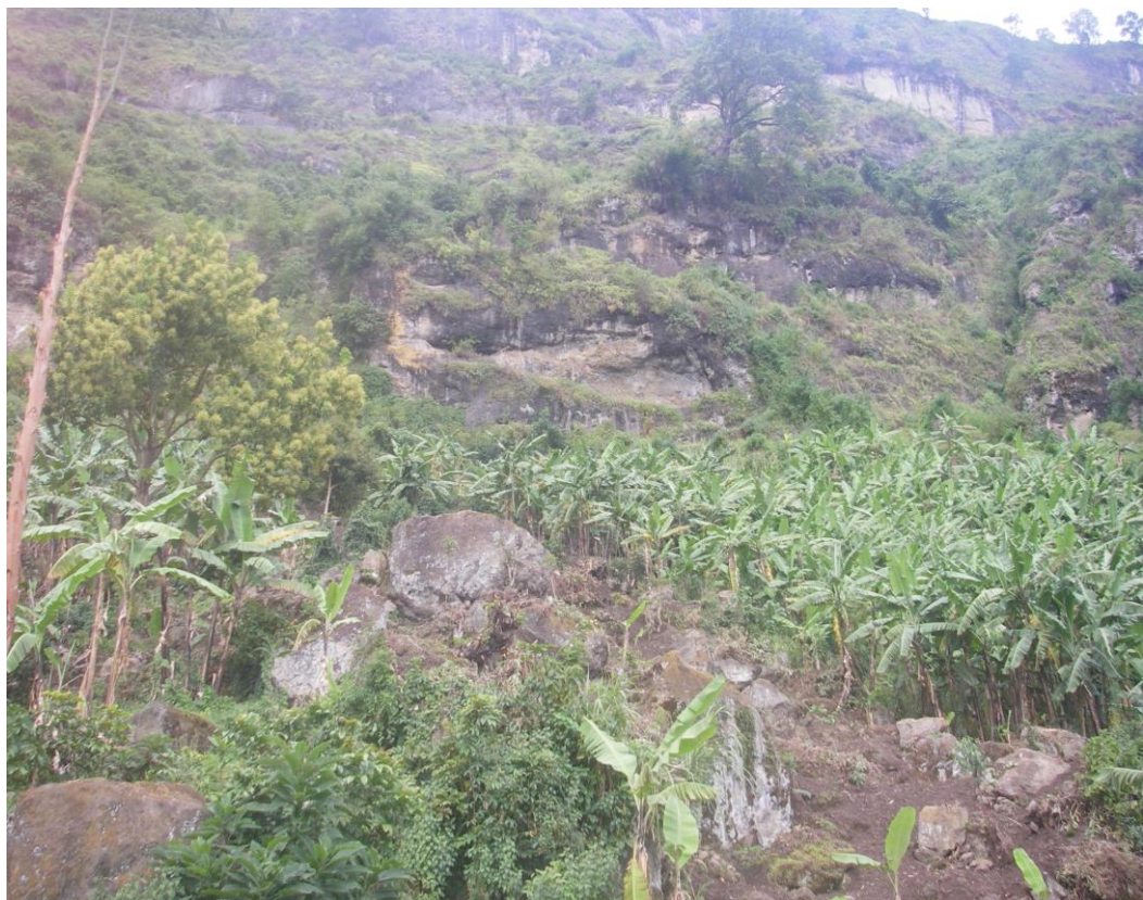
Plate 5.5a: A debris slope vulnerable to rock fall from an adjacent scarp face (Namudongo- December 2009)
