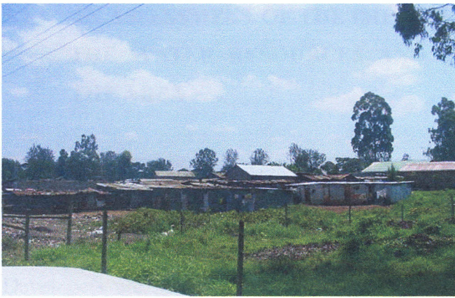
Plate 4 Poorly planned high density housing in Kuwinda Settlement (Source: field survey, 2010)
