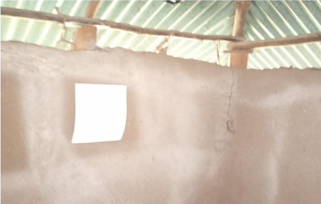
Figure 1.2 : Sampled dwelling revealing the gap (reru) between the roof and the wall the smeared wall
