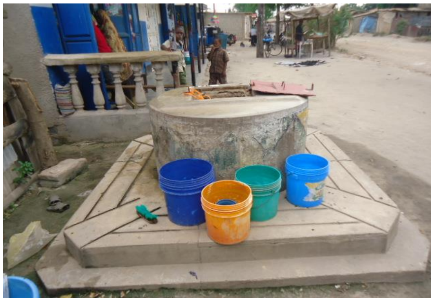
Plate 4.5: Covered Deep Well at Tabata Liwiti Area ( Field Survey, 2012 )
