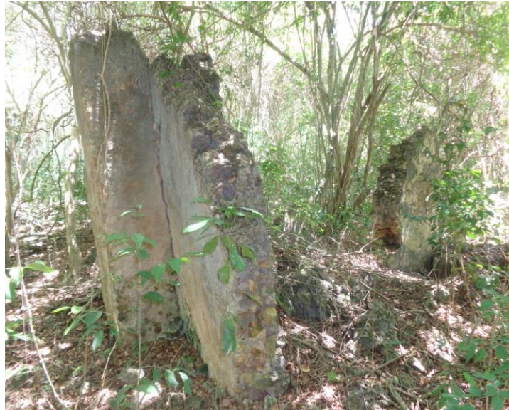
Plate 3.1: Some of the collapsed wall structures in the forest Source: NMK Gedi
