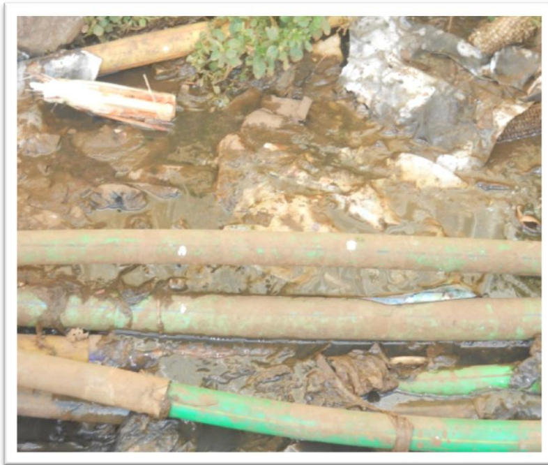
Plate 5.3: Water Pipes in the Drainage
