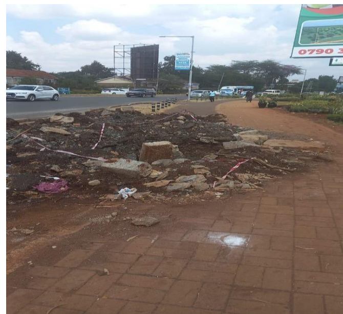
View the storm water management system. Source: Authors, 2025
