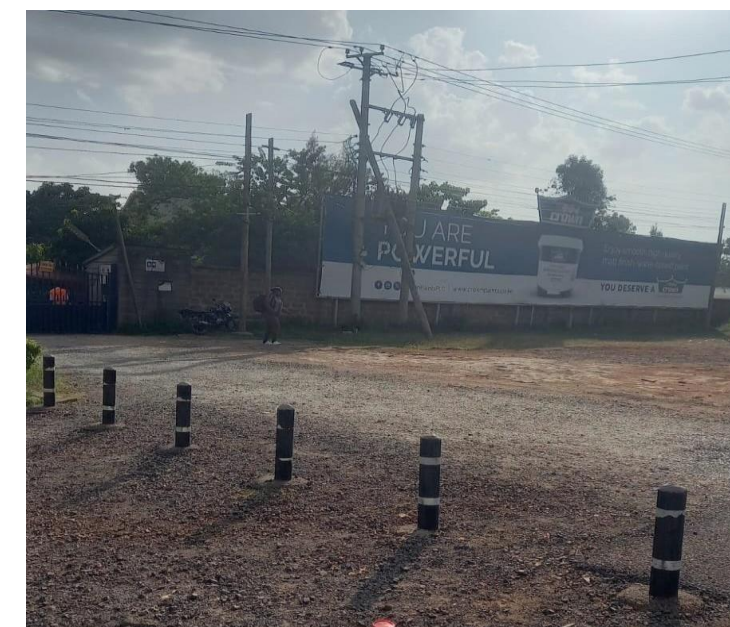
Current state of the access road to Impala club. Source: Authors, 2025
