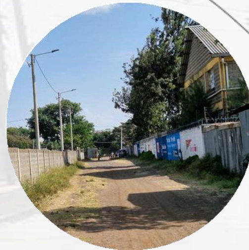
Combined Sewer and Storm Water Drainage
