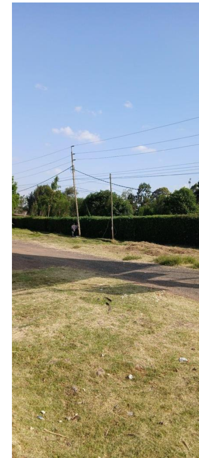
View of the electricity supply And the back up generator Source: Authors, 2025
