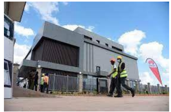
The Data Centre at Konza Konza Technopolis, 2024
