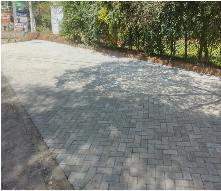
A cabro paved road in Nairobi. Source: Propavers, 2023
