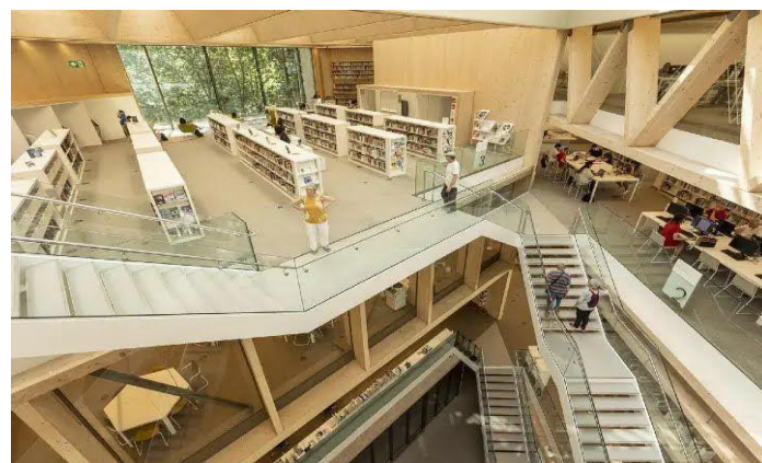
Library interior showing extensive use of wood Source: Metalocus
