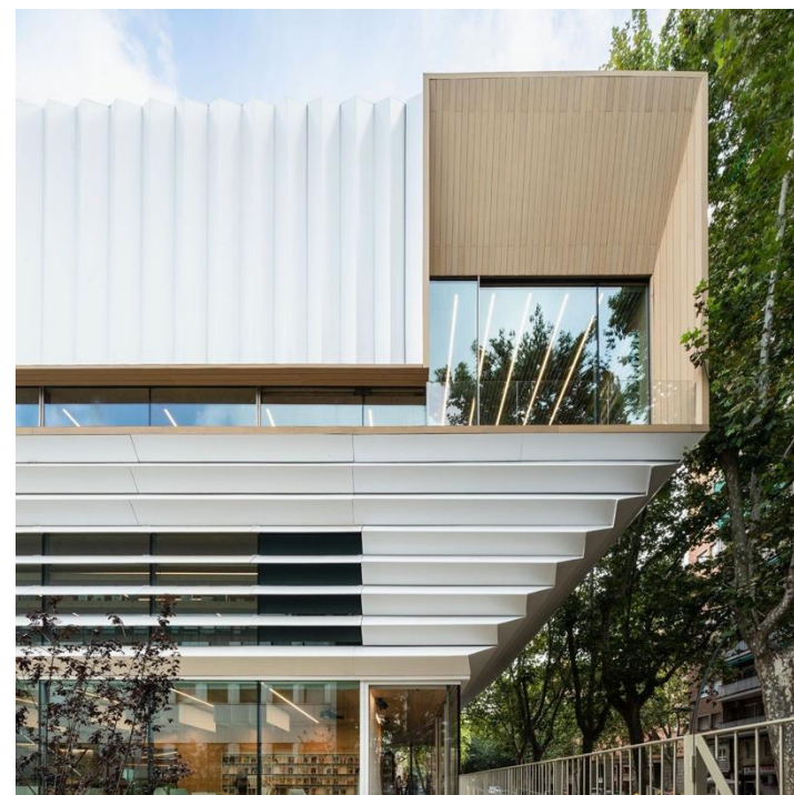
The two images above show the bay windows on the Library's facade. They provide natural lighting as well as promote connection to the external environment. Source: Metalocus official website
