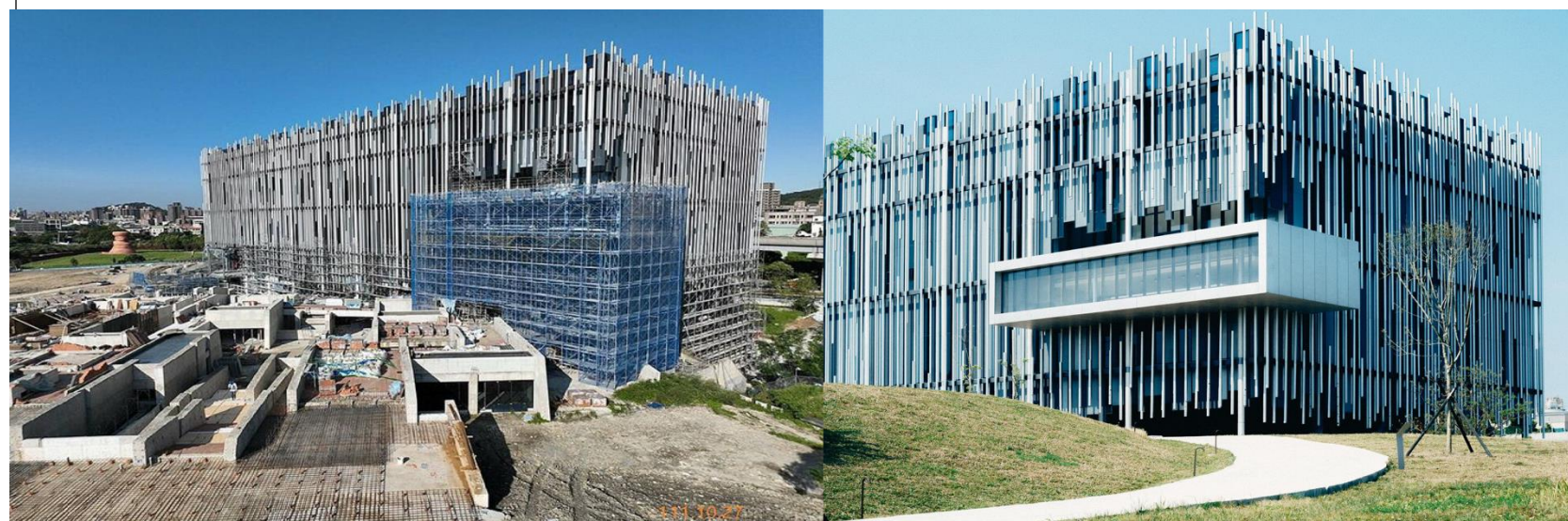
Exterior view during construction
