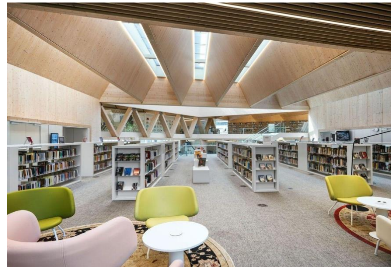
Photo : Triangular Void acting as a solar chimney, Gabriel García Márquez Library Source : Jesus Granada
