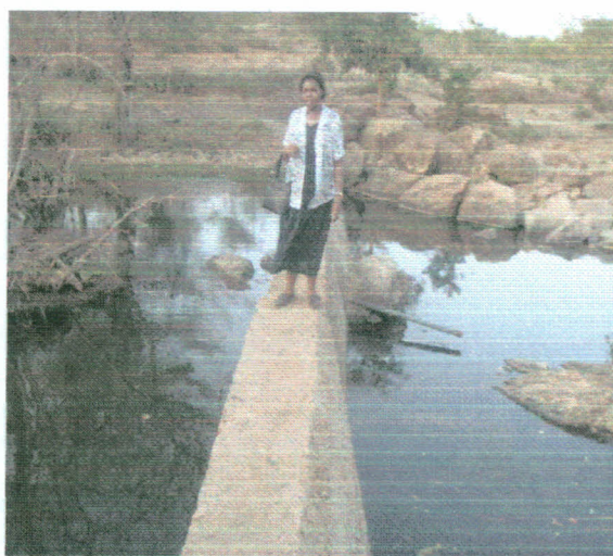
Dam under construction
