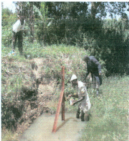
Rehabilitation of RGS along ENA River in Mbeere)
