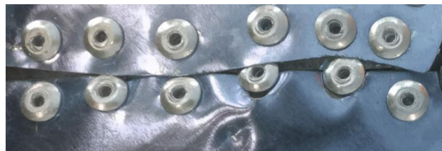
Riveted metal sheet
