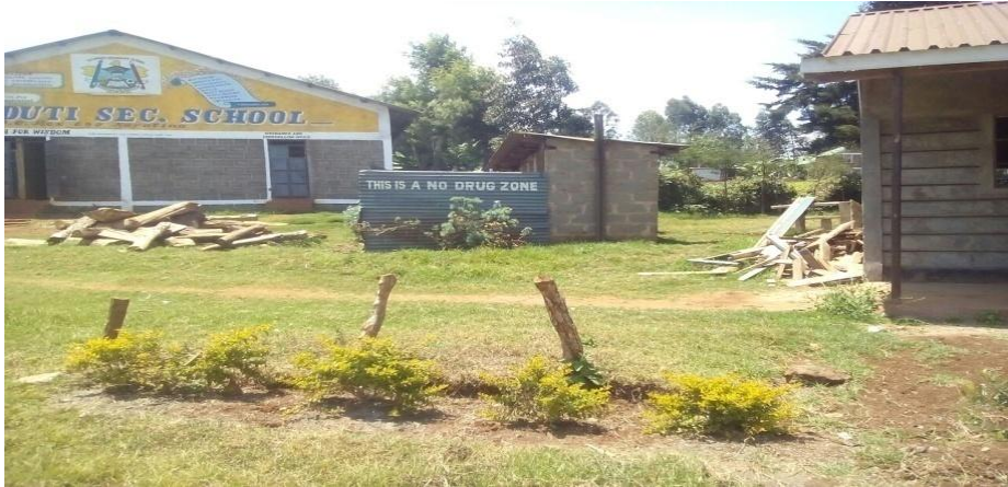
Figure 4.14: An Example of Inappropriately Constructed Pit Latrines between Classrooms and Administration Block
