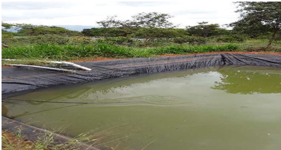
Plate 4.1: Water pan constructed by WVK in Kanzokea
