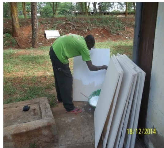
Plate 37: Applying second coat Source: Researchers photo
