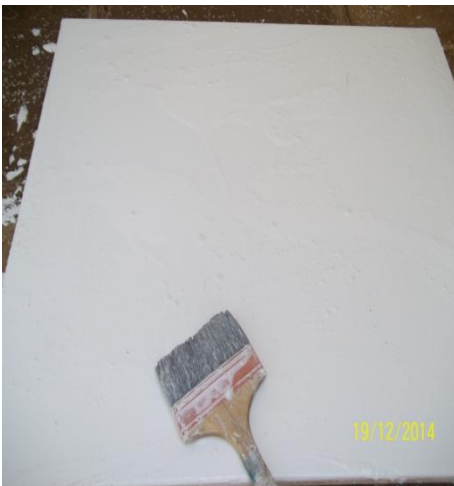
Plate 36: Applying Second coat Source: Researchers photo
