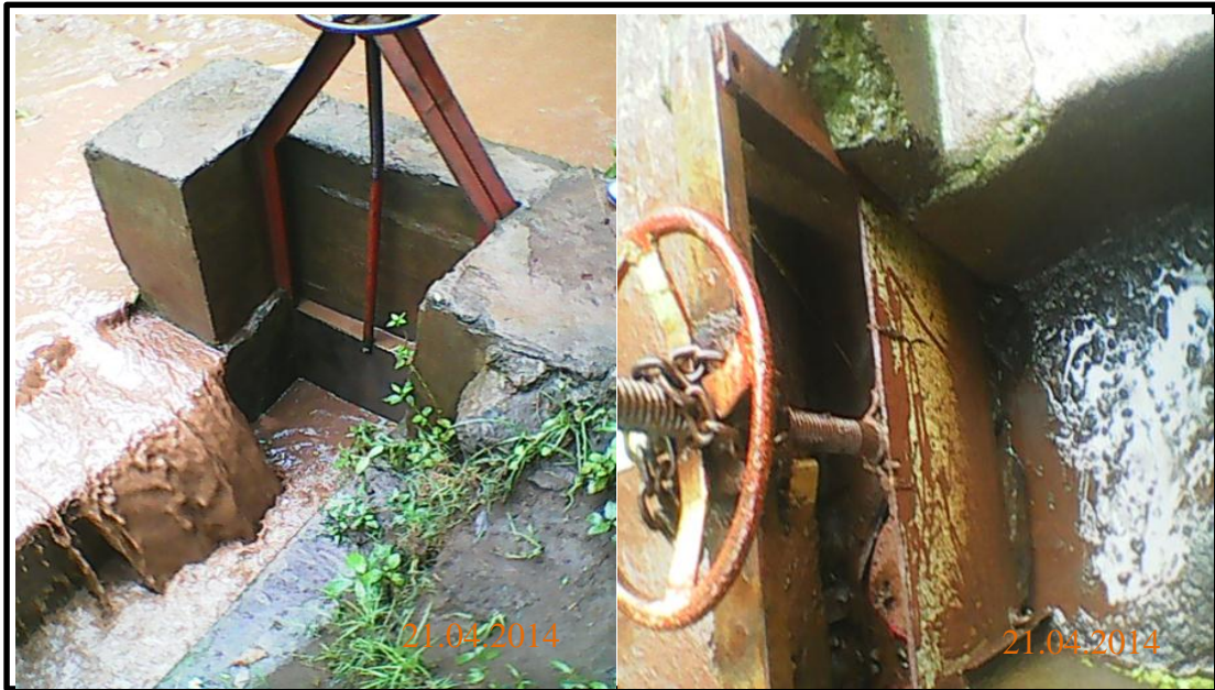
Plate 4.6: Closed gates during rainy season in Kiladeda river (Source: Author, 2014)
