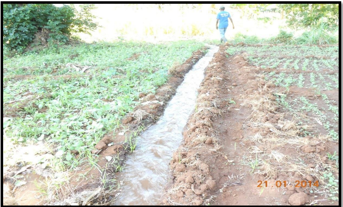
Plate 4.4: Existing tertiary furrow in Kiladeda sub catchment (Source: Author, 2014)
