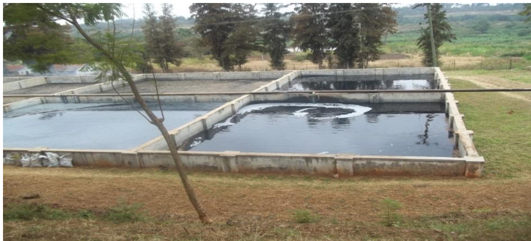
Plate 4. 1: Wastewater treatment plant (WWTP). Picture for noon 24 th July 2013.
