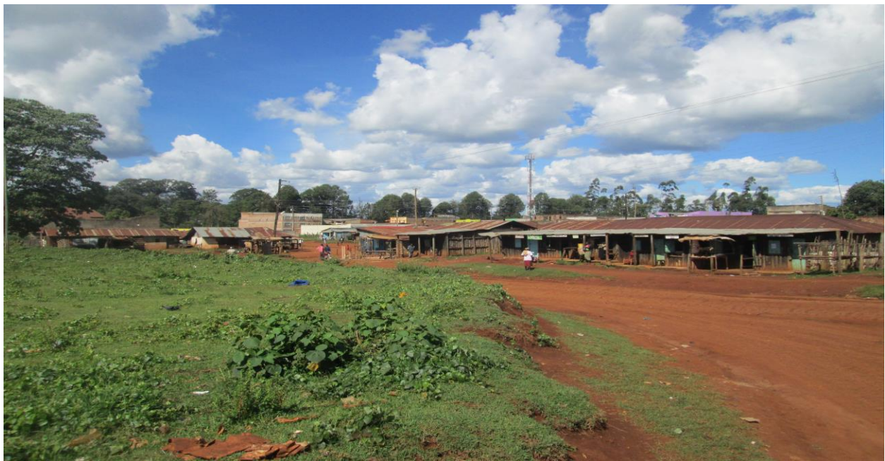
Plate 5: Dilapidated houses and section of open space
