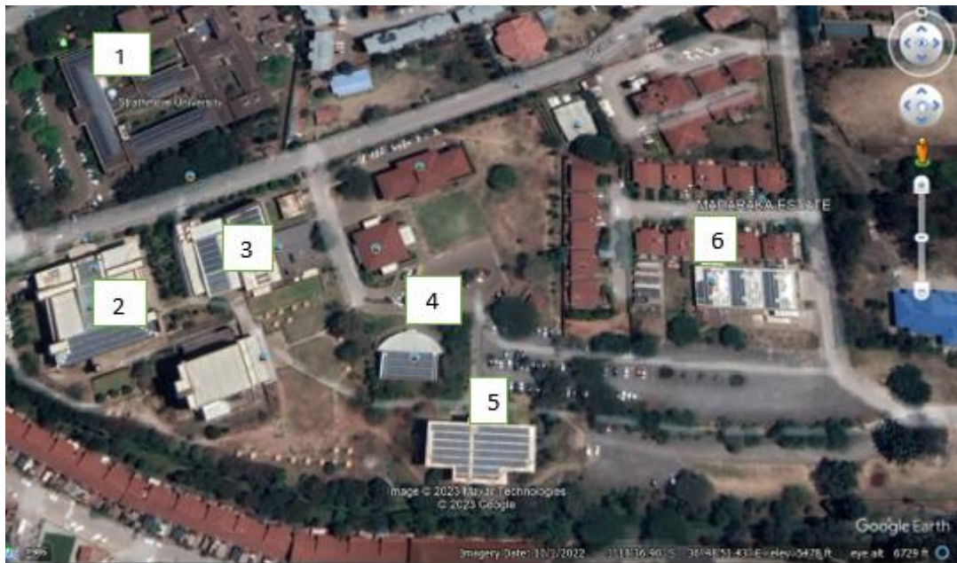
Figure 4.1: Solar PV system spread on Strathmore University building rooftops (Google Earth, 2022)
