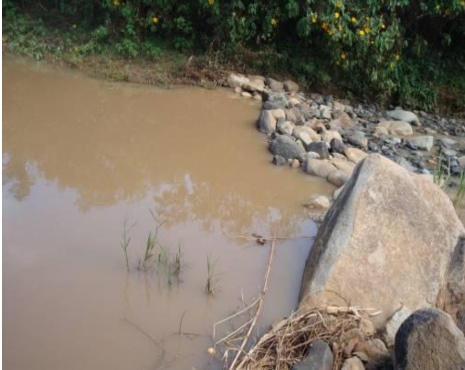
Plate 8. Boulder weir at Upper Awach-seme site AS1 showing a pool formed a head of the weir.
