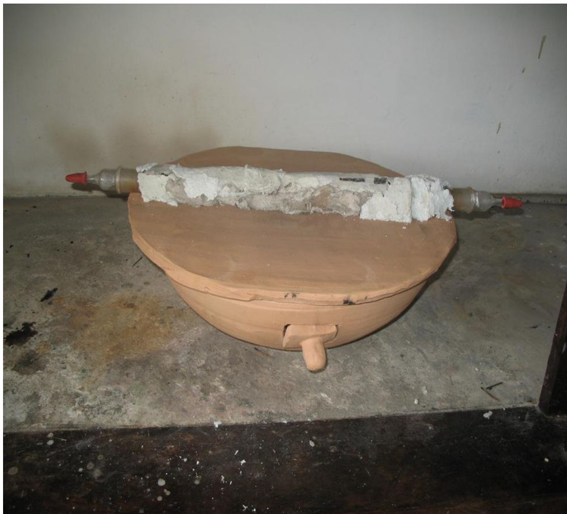
Fig. 3.9 Glass column covered with asbestos
