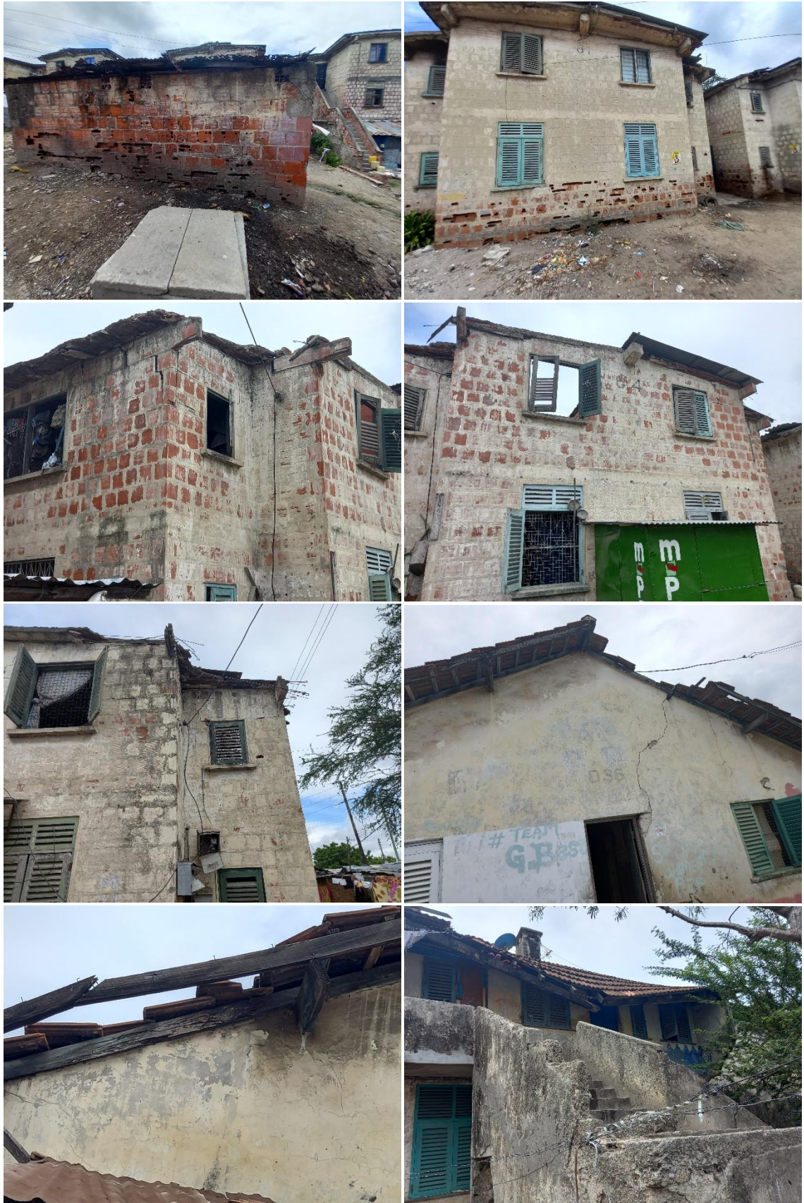
Figure 4.2 Proposed houses to be demolished for AHP
