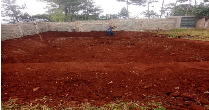
Photograph 3.1: Excavation of ESP funded fish ponds at Mathira constituency
