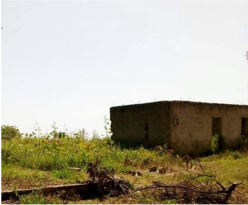
Plate 4: The side view of demolished house
