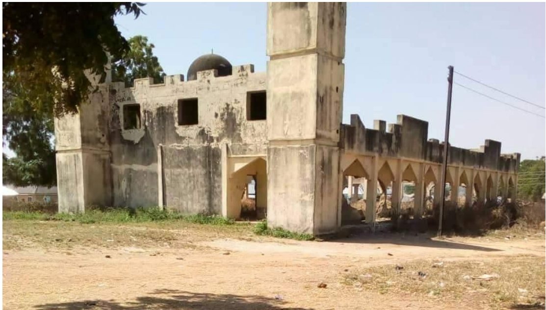
Plate 3: The side view of demolished Mosque Source: Researcher (2020).
