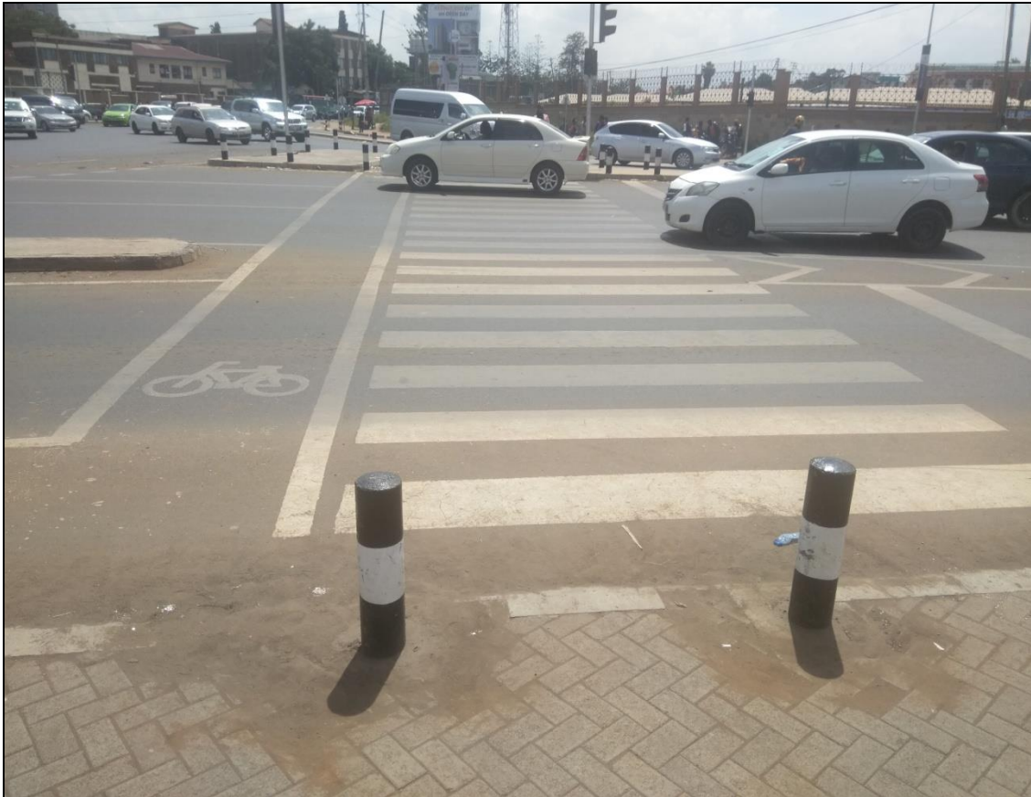
Plate 4. 3. Clearly marked pedestrian together with bicycle crossing on Ngong' Road in Nairobi
