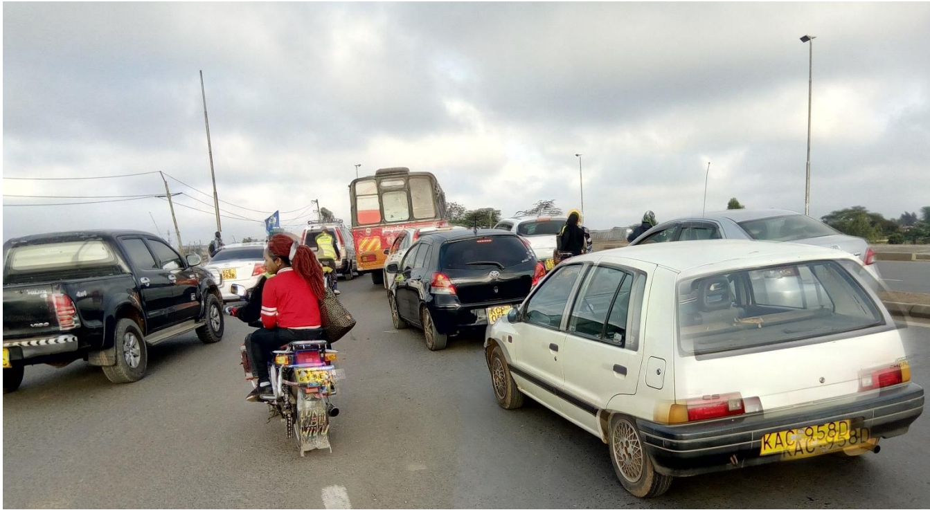
Two roads with two lanes from Manyanja and Lungalunga each joining Jogoo road's two lanes is a form of bottlenecking
