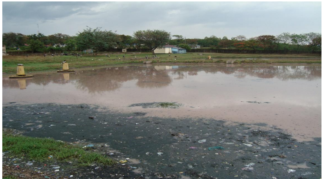
Plate 3.7: Sewage treatment plant machines in a dilapidated condition next to site L5.
