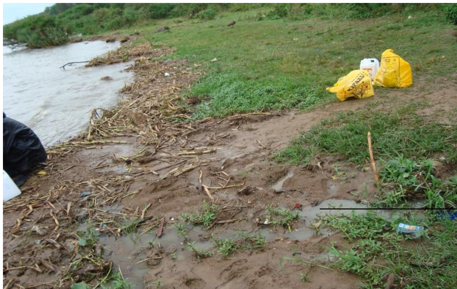
Plate 3.9: Sewage effluent discharging into the lake next to site L6.
